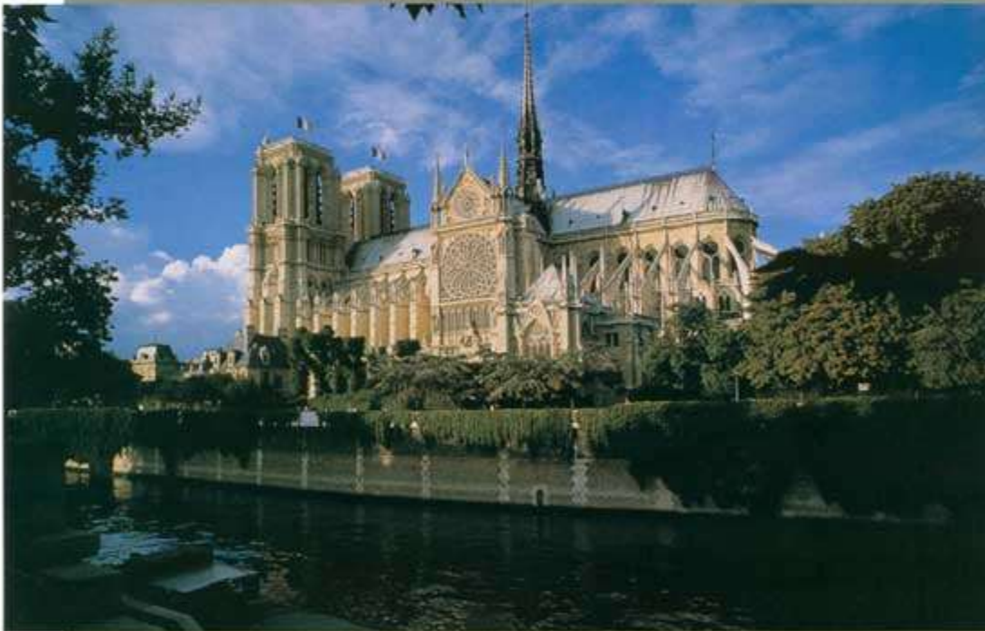
16-22. Cathedral of Notre-Dame, Paris. Begun 1163; choir chapels 1270s; spire 19th-century replacement. View from the south
